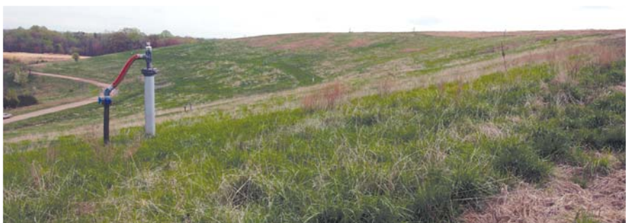
Methane from the Sandy Hill Landfill in Bowie, Maryland had been burned off in a flare until NASA officials at the Goddard Space Flight Center built an on-site purification plant. Wells (above) now draw methane out of the landfill, moving it to the processing plant (lower right) for renewable power generation.
