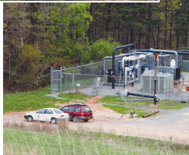
Methane from the Sandy Hill Landfill in Bowie, Maryland had been burned off in a flare until NASA officials at the Goddard Space Flight Center built an on-site purification plant. Wells (above) now draw methane out of the landfill, moving it to the processing plant (lower right) for renewable power generation.
